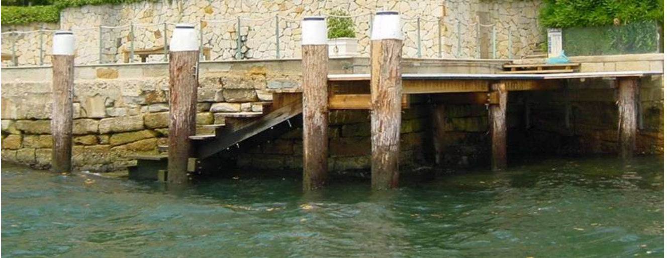
Harbour wharf and Seawall engineering and construction
