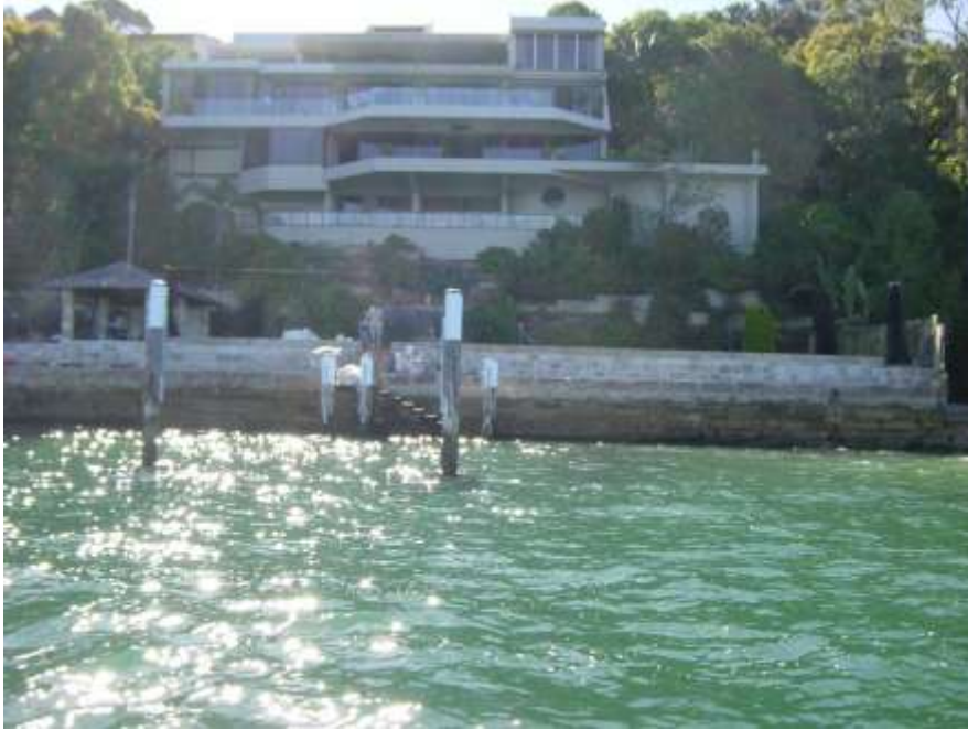
92 Wolseley Road Point Piper Seawall construction and Jetty repair
