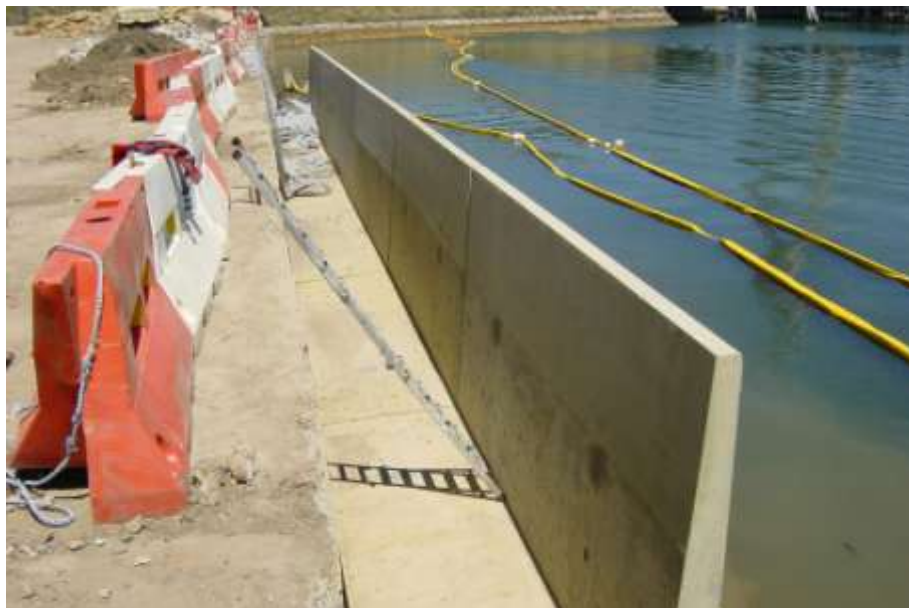
Precast panels in place
