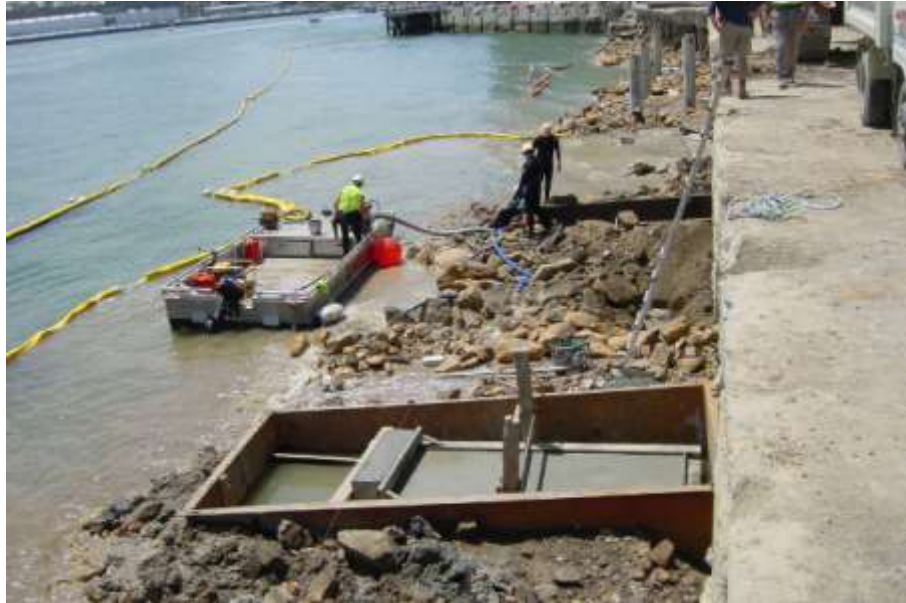
Cofferdams used for headstock construction
