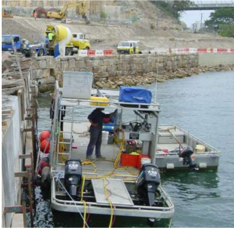
Diving operations and sandstone seawall
