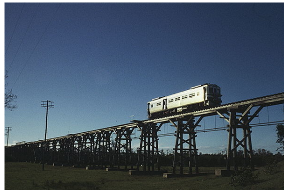
RM 1901 crossing the Splitters Creek bridge ~1989
