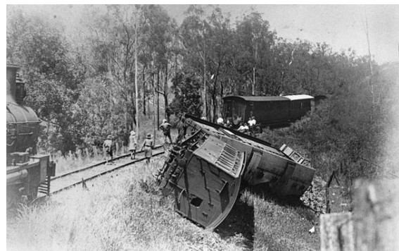
Railway carriages derailed at Gillen Siding on the Mount Perry branch line, 1924
