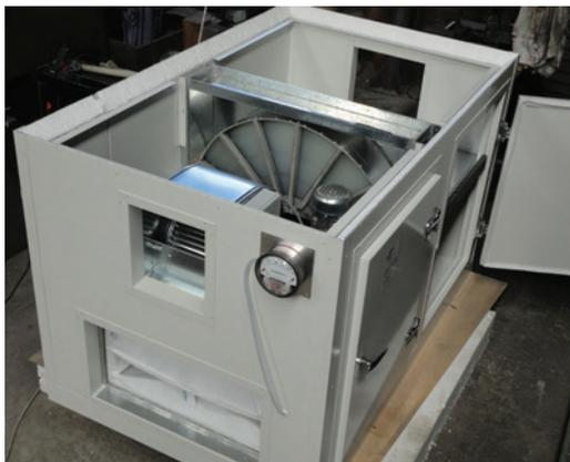
A typical AHU with a Mylar wheel installed at the Oakridge Estate Winery in the Yarra Valley, Victoria.
