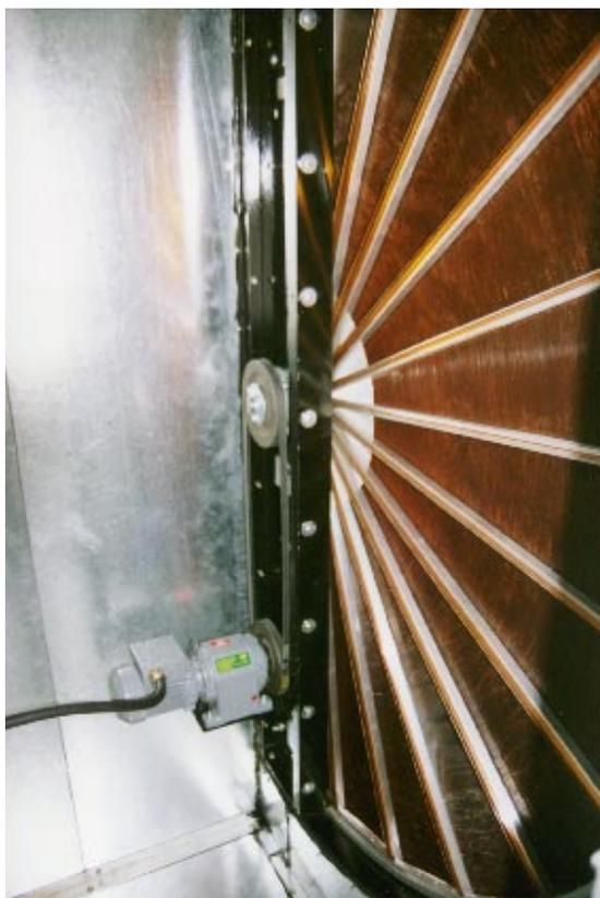
The interior of the rotary heat exchanger as used in the adhesive labelling dryer at Jac Pty Ltd.
