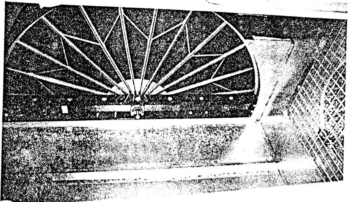
THE ROTARY HEAT WHEEL INSIDE THE PLENUM CHAMBER WHICH SEPARATES THE EXHAUST FROM THE HEATED FRESH AIR
